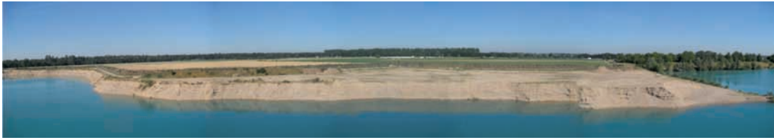
Fig. 3: Steep embankment being dredged against
